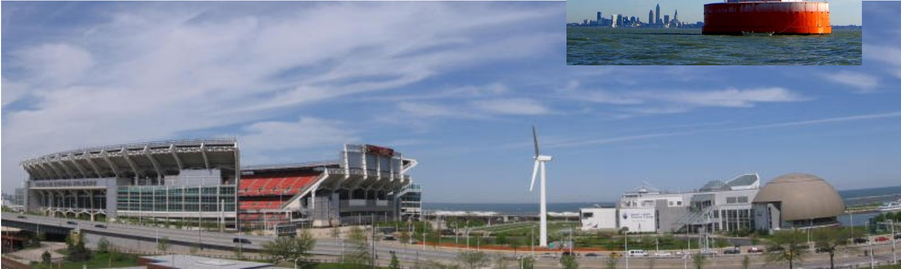
225 kw turbine on Lake Erie waterfront, downtown Cleveland
