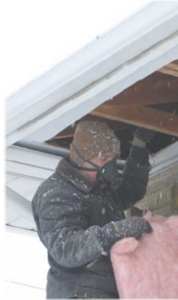
Right: a local contractor installs traditional insulation under the roof eaves of a Independence home. By insulating the home here, it will prevent the heat from escaping, thus providing a warmer more efficient home for the participant.
