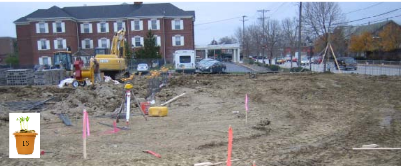
City of Shaker Heights. The Library Court site as it appears during construction.
